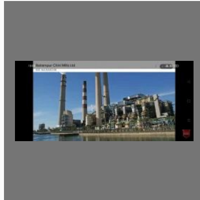
Commercial Electrical Contractor Services
